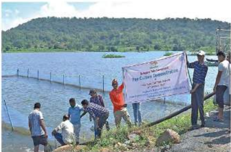
CIFRI HDPE pen installation in Ukai, Gujarat
