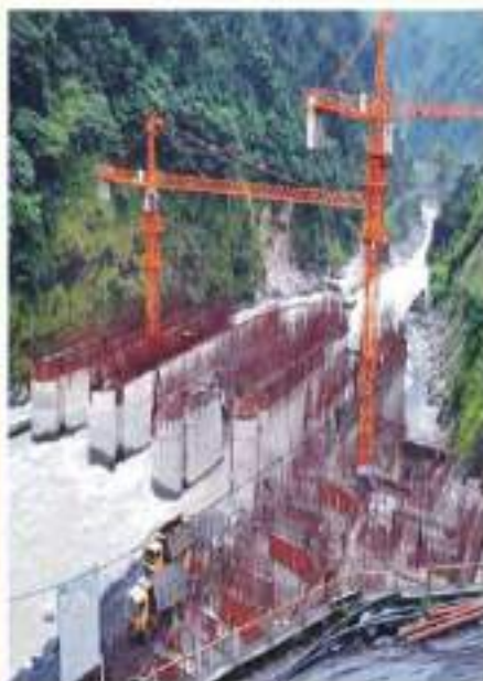
Dam under construction on River Rangit
