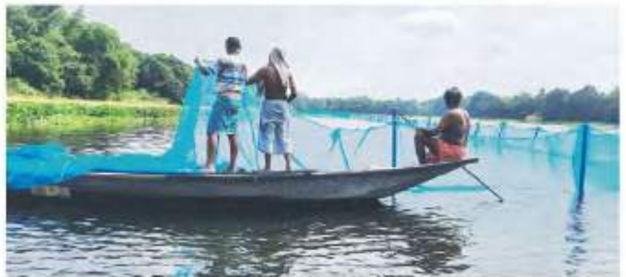
Installation of pen in progress
